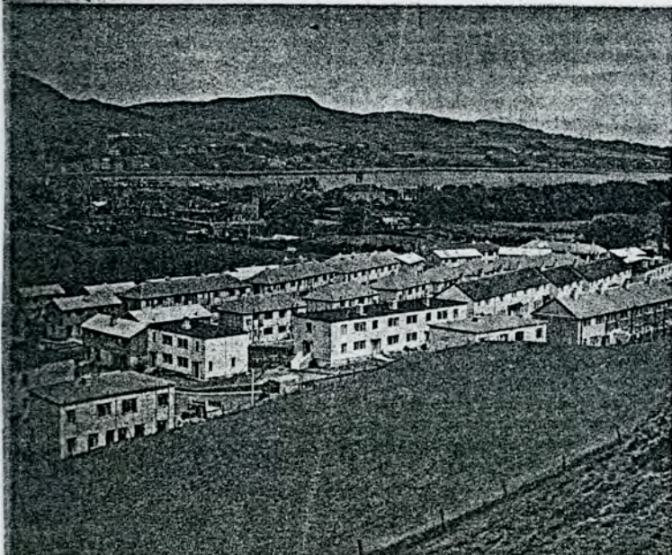
Half of these new houses going up on the Crosshill-Meadows housing estate are reserved for incoming miners—many from Lanarkshire's redundant mines
