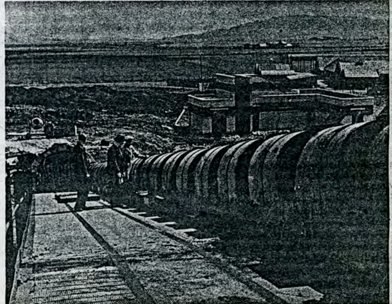
From the mine entrance rises the main drift conveyor to the screens. In the background is the country over the coal basin to which Argyll is heading
